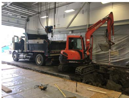
Installation of four new bus lifts at the Transportation Center.
