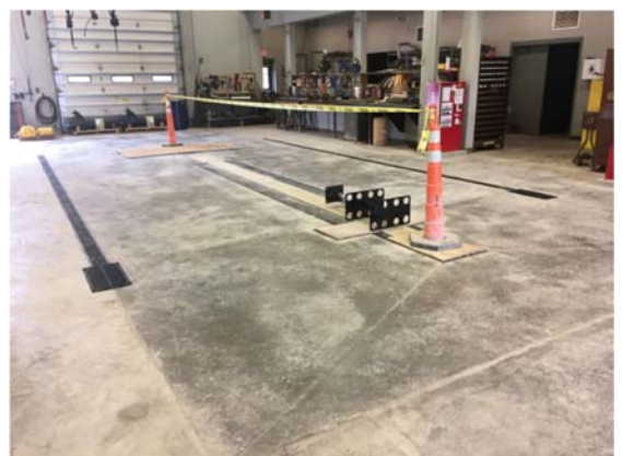
The final bus lift installation nearing completion
